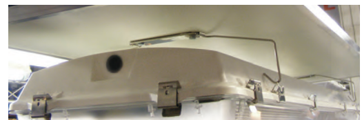
1.25" between ceiling and enclosure
