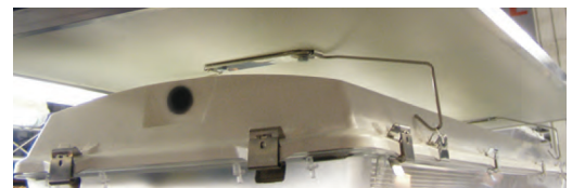
1.25" between ceiling and enclosure
