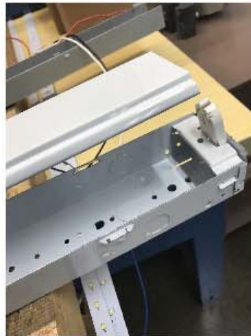
Remove Ballast Cover
