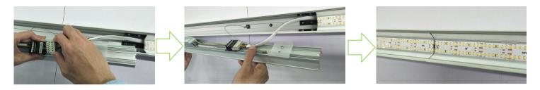
A12. Install diffusers (Keep about 1.5mm space between diffuser and end-cap on last two ends)
